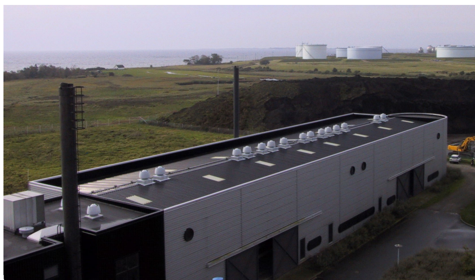
Existing reactor housing at Stignæs Industripark; Denmark
